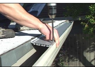
10. Drill in three screws in the front. This procedure can be performed before the caulking step in number 9 above if you wish. That's all there is to it.
