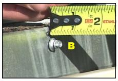
5. Drill two screws in the back of the fascia for holding up the piece of Gutterglove you just cut. You may also use three screws in the back if you wish. Leave the screws about 1/2 of an inch backed out (Insert B). Gutterglove should be able to rest more than adequately on this.
