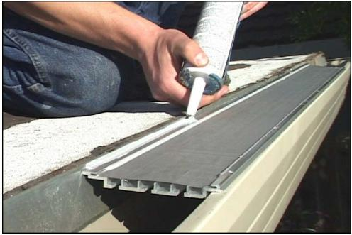
9. Apply caulk in the back edge between Gutterglove and the roof.
