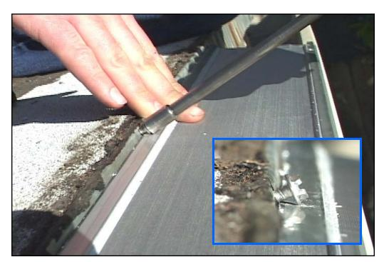
8. Drill two screws into the upper portion of the fascia to assist in holding down Gutterglove.
