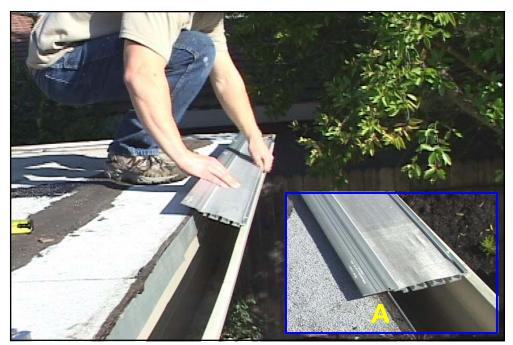
1. The back wing rests over the roof portion (Insert A.).
