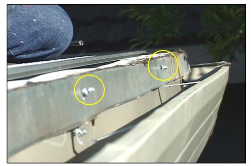
6. Two screws for supporting Gutter-glove.
