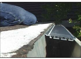
7. Gutterglove rests neatly on top of the gutter and about 1/4 inch lower than the roof.
